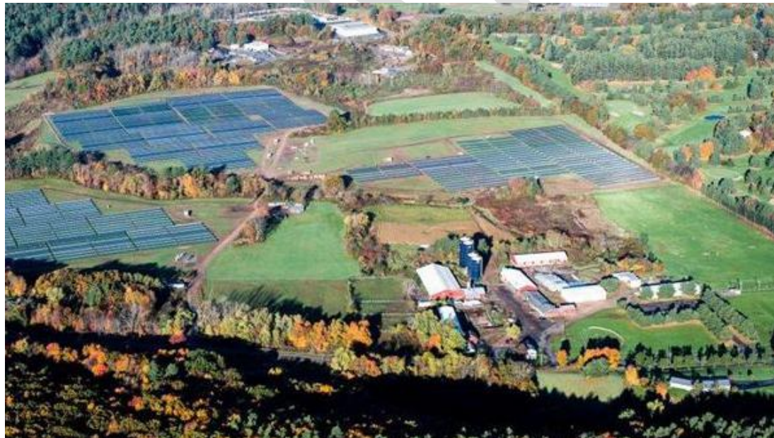
Solar Array on Route 83
